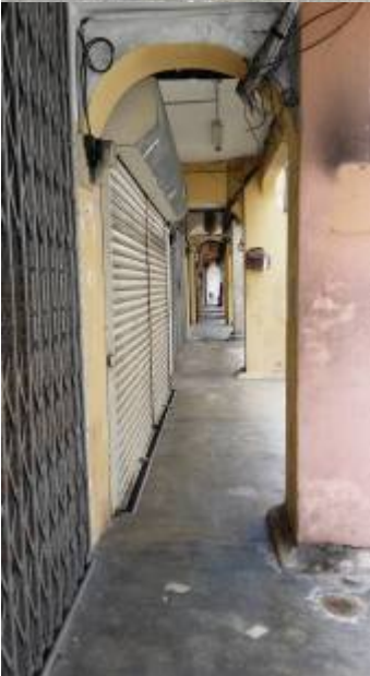
“While walking back to Kajang Heritage Centre from Kedai Buku MakAli, took a photo of the narrow five-foot way linking old shophouses along Jalan Tengah. The row of relatively smaller shops are supposed to be the earliest brick shophouses in Kajang Town. History record says that the first batch
